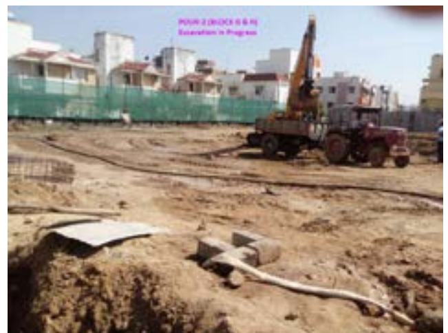
Excavations Process of Block G and H
