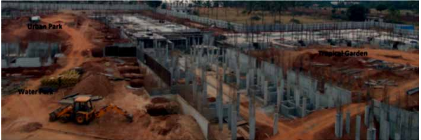
Arial View of the project site
