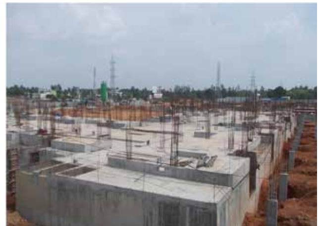
Completion of Basement for Villas
