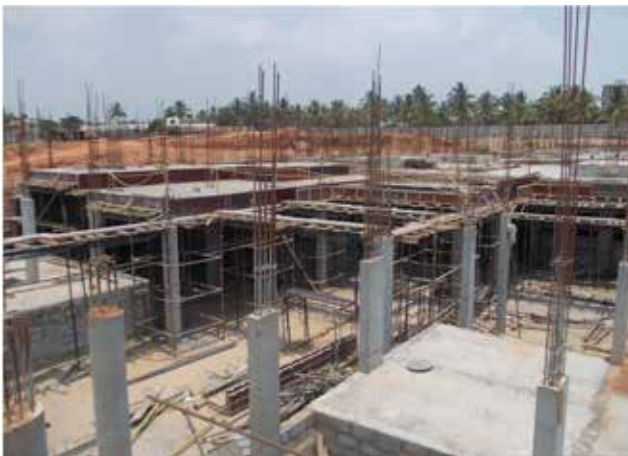
Super structure work of Villas in progress
