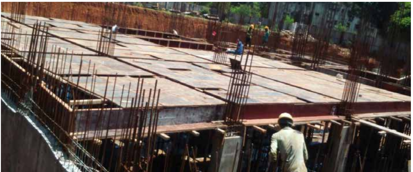
Ground Floor slab framework in progress
