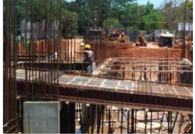
South side ramp from UB floor level to stilt floor level works in progress
