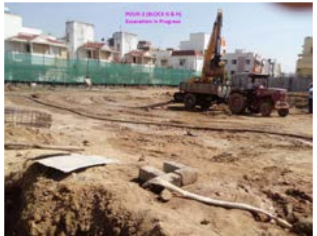
Excavations Process of Block G and H
