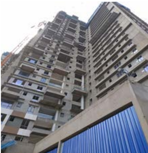
Photograph: Tower B
