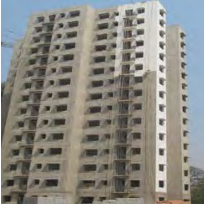
(i) Hiland Greens Phase I, painting work in progress
