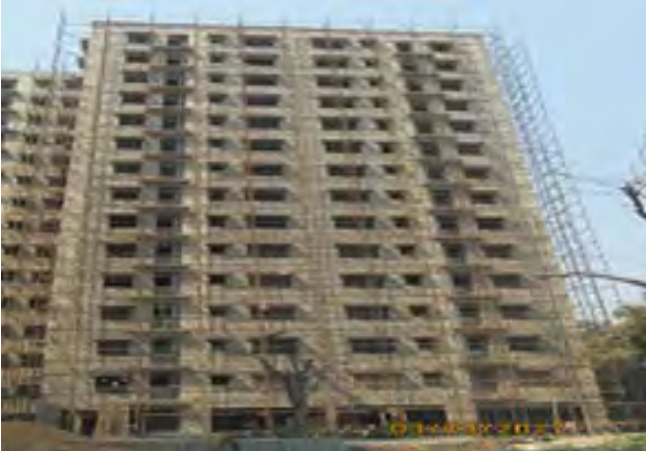
(ii) Hiland Greens Phase II, outside casting work in progress
