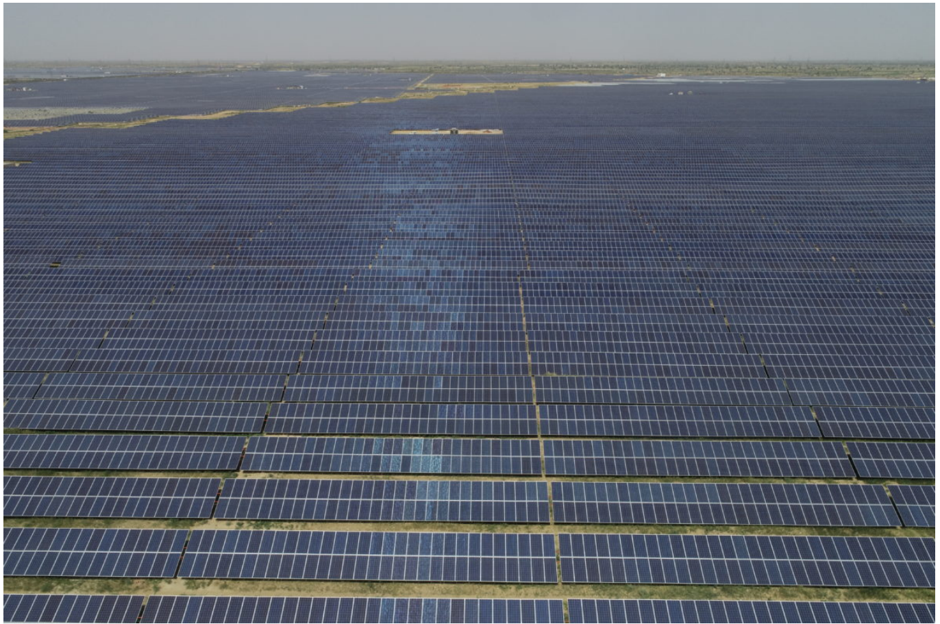
Acme Solar's Bhadla plant in Rajasthan
