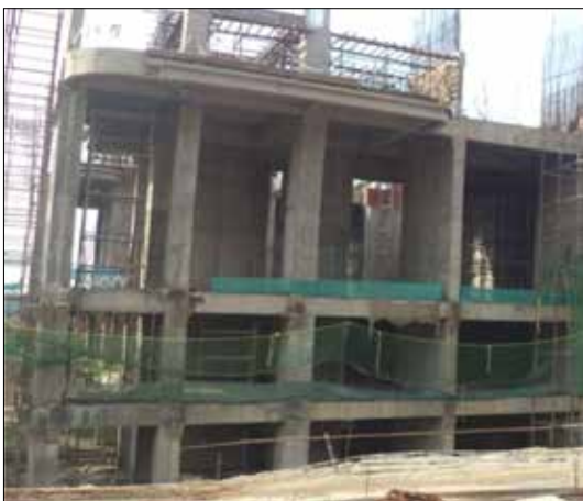
Tower 5 :- Raft, 2 Basements completed, Ground floor slabs completed
