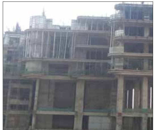
Tower 4:- Raft, 2 Basements completed, fourth floor slabs completed
